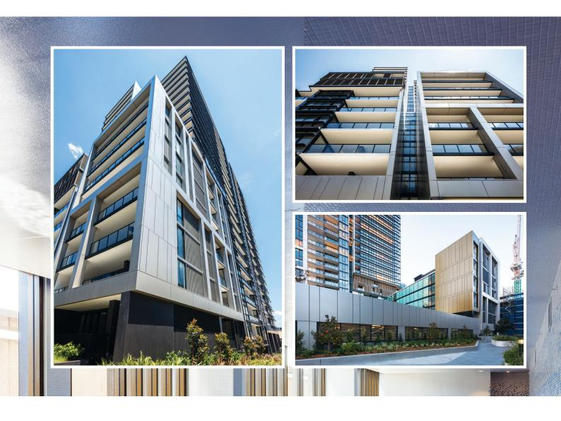
More than 7,000m<sup>2</sup> of aluminium composite panels were installed for the Savannah project at Sydney's Wentworth Point. Based in Chipping Norton, Sydney, Australian Cladding Specialists manufactured the panels in their 1,500m<sup>2</sup> factory featuring the latest high-tech machinery.
