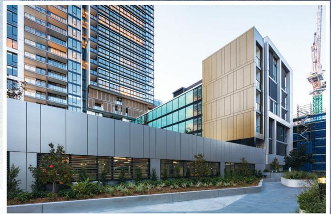
**More than 7,000m<sup>2</sup> of aluminium composite panels were installed for the Savannah project at Sydney's Wentworth Point.** Based in Chipping Norton, Sydney, Australian Cladding Specialists manufactured the panels in their 1,500m<sup>2</sup> factory featuring the latest high-tech machinery.
